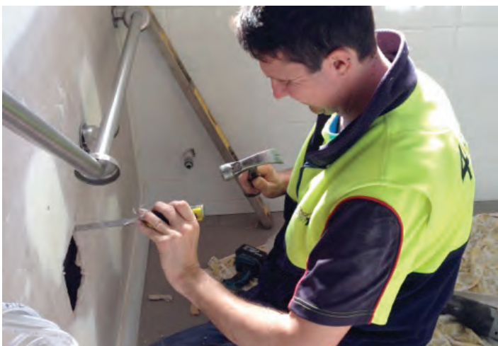
UNDER CONSTRUCTION: Emily Cottage bathroom
