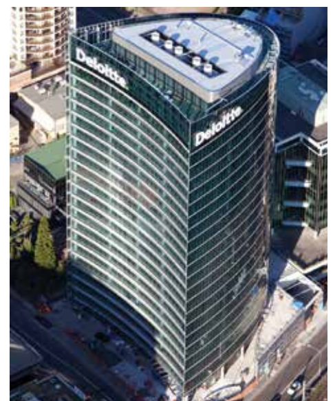
Eclipse Office Tower, Parramatta by Leighton Properties
