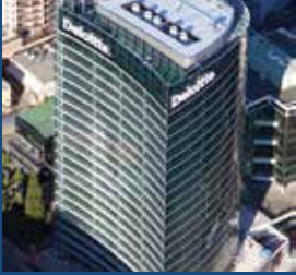
Eclipse Office Tower – Parramatta by Leighton Properties
